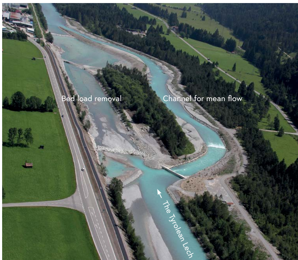
Bed load excavation facility Höfen-Hornberg: A new channel for mean flow was constructed in parallel to the bed load trap. It serves to transport the necessary, although reduced, amount of bed load downstream.
