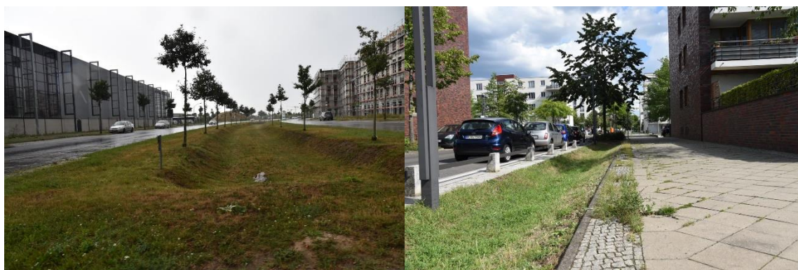
Fig. 10. Infiltration ditch as an example of retention areas which should be considered in local spatial development plans (phot. I. Lejcuś)
