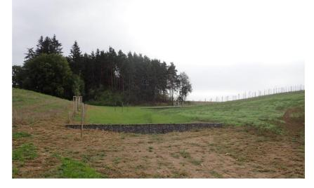
Figure 14: Upstream view of the barrage realized on an agricultural field (source: VÚV TGM, v.v.i.).
