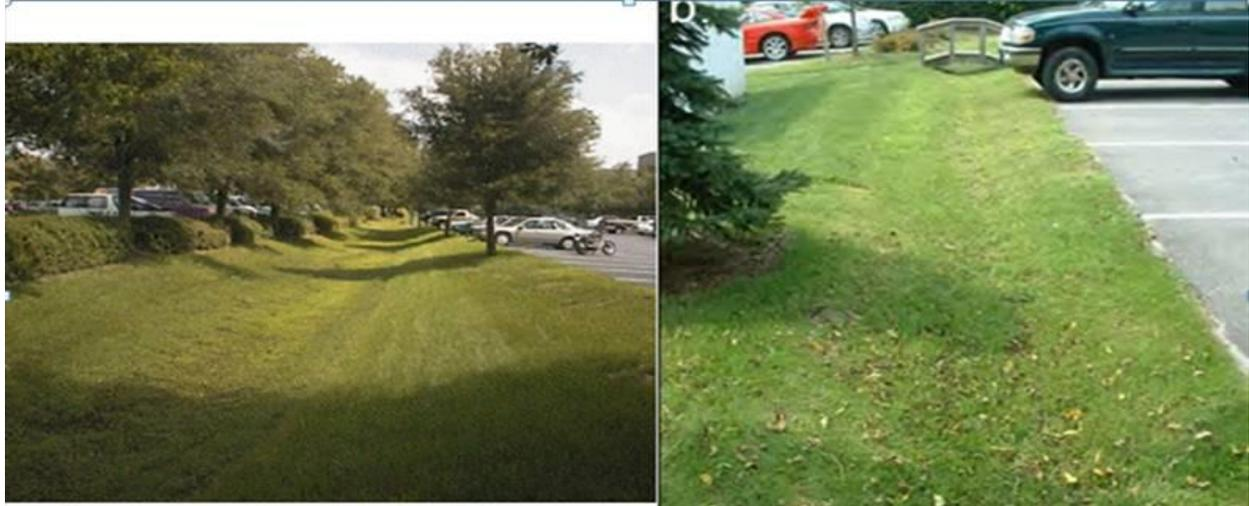
Figure 29. Grassy ditches and swales (source: RBMP, Urban rainwater management guide, 2015)
