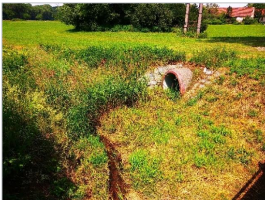
Relief pipe at culvert (source: The Region of South Bohemia, The Section of Territorial Planning)
