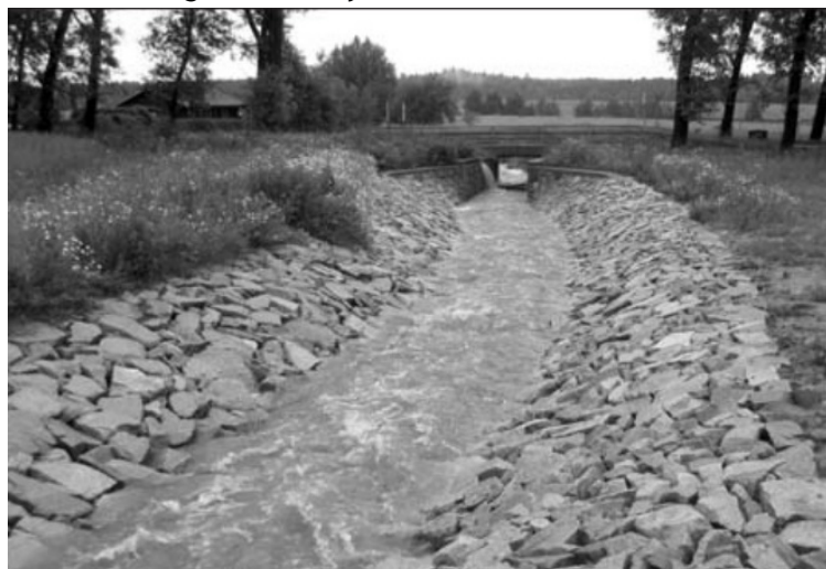
Channel filling durin heavy rain event in 2009:
