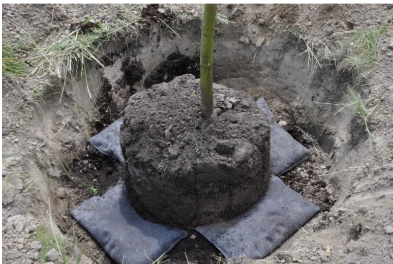
Water absorbing geocomposite (GSW) under tree and on the embankment (good condition of plants has anti-erosion effect) Source: K.Lejcuś
