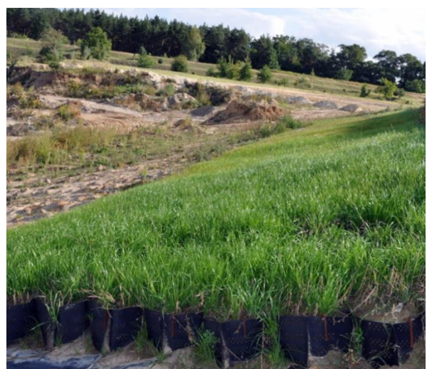
Water absorbing geocomposite (GSW) under tree and on the embankment (good condition of plants has anti-erosion effect) Source: K.Lejcuś
