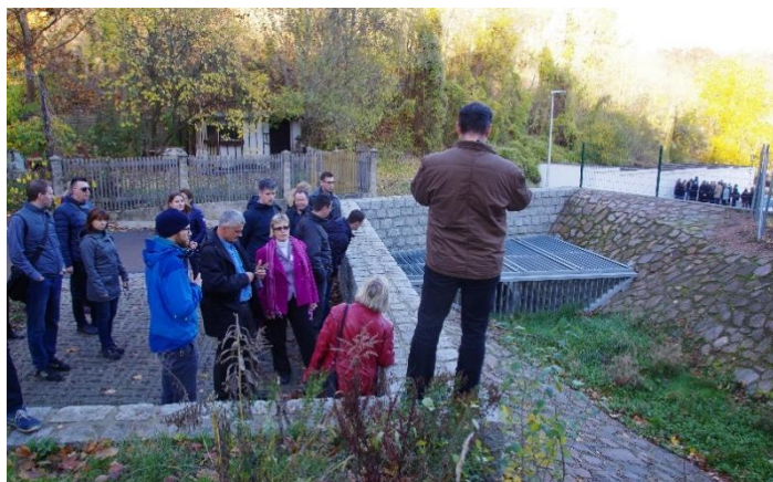
Renewed pipe and inlet rake at the lower part of the stream course Source: Sabine Scharfe, LfULG
