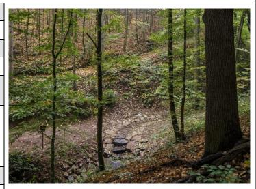
Bank reinforcement in a bump curve of the brook "Kirchsteigbach" Source: P. Voigt
