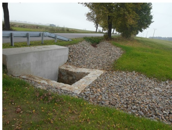
Culvert under the road
